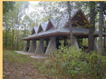
Existing picnic shelter
