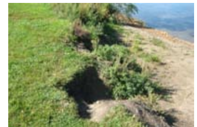
Before - Eroding Shoreline Lake Volney Shoreland
