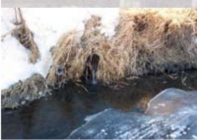
Straight pipe outlet from historic trench into Straight River.
