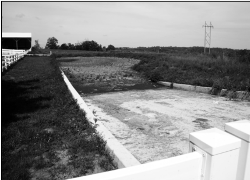
The newly constructed manure storage pit can hold 500,000 gallons of manure.
